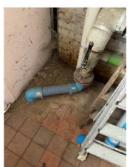
Incoming water main in boiler room connected to old galvanised pipework
