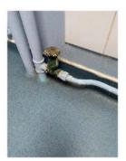
Example of old pipework and valves with pipework run in floor
