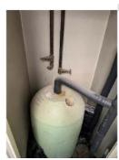
Example of dead legs in cold water down system on old galvanised pipework
