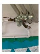
Example of use of percussion tees where additional heat emitters have been installed to original pipework
