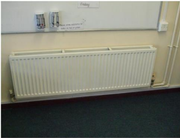
Picture 7- Block 11 Radiator with TRV in satisfactory Condition (B4). Pipework to be replaced with new (D1)
