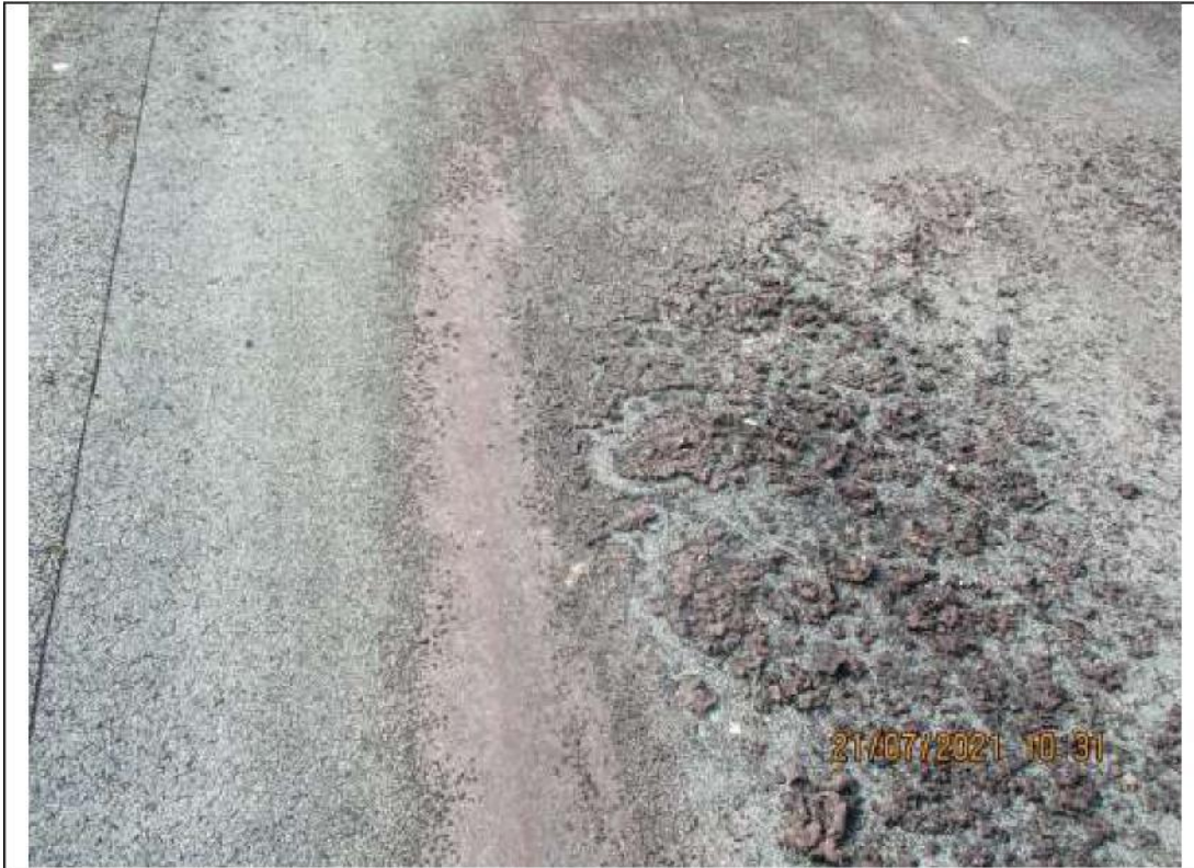
39) Higher level roof to KS1 area.
