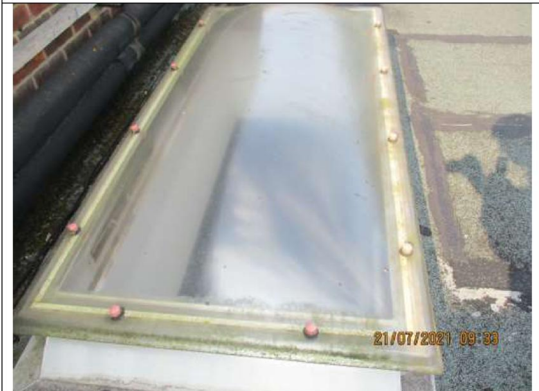
6) Typical roof light.
