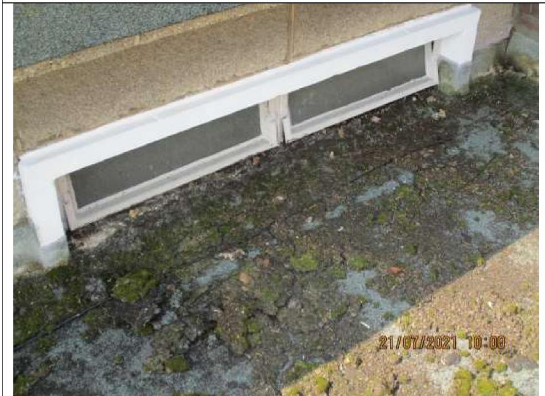
26) Low level windows to roof adjacent to the nursery.
