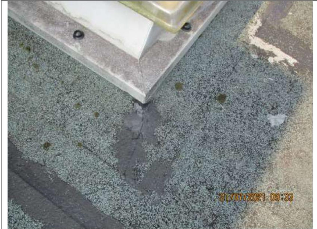
5) Patch repairs to upstand detail to roof light.
