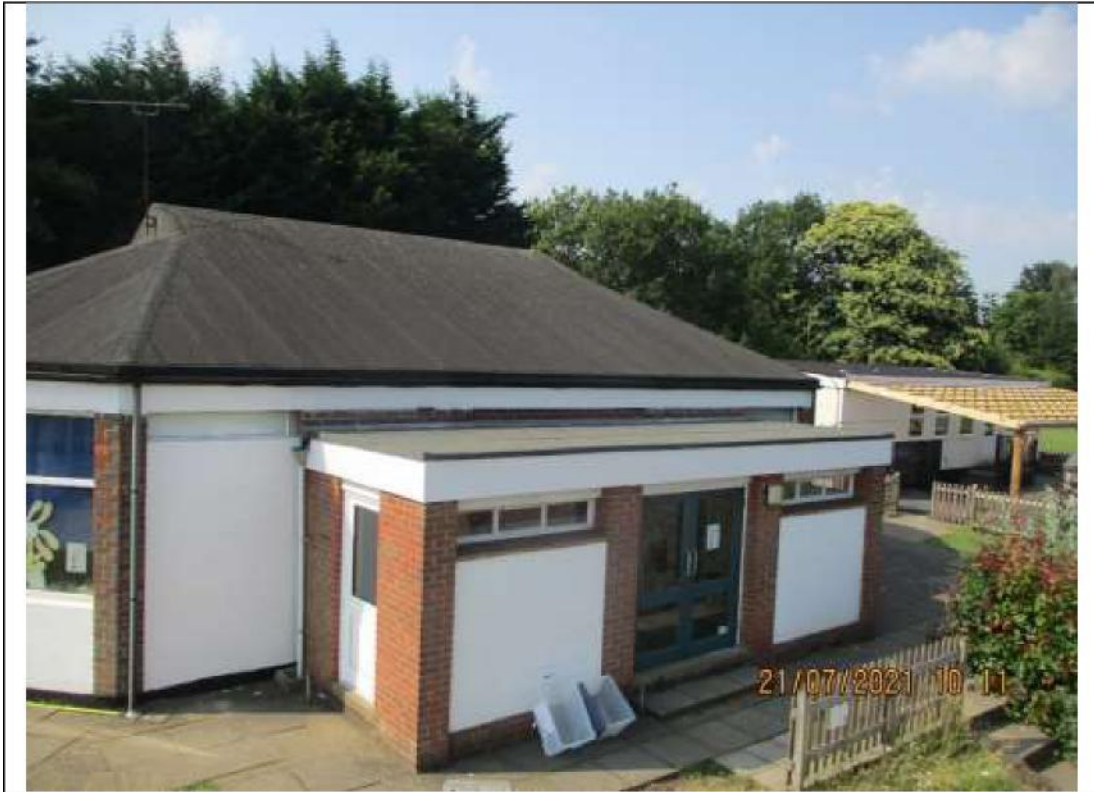
31) Roof above Year 5/6 block.
