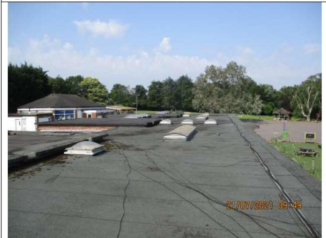
16) Roof above KS2 area.
