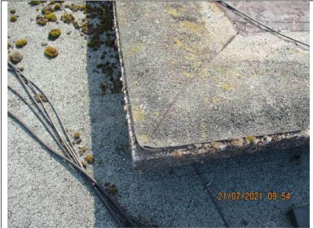
21) Patch repairs to roof above KS2 area.
