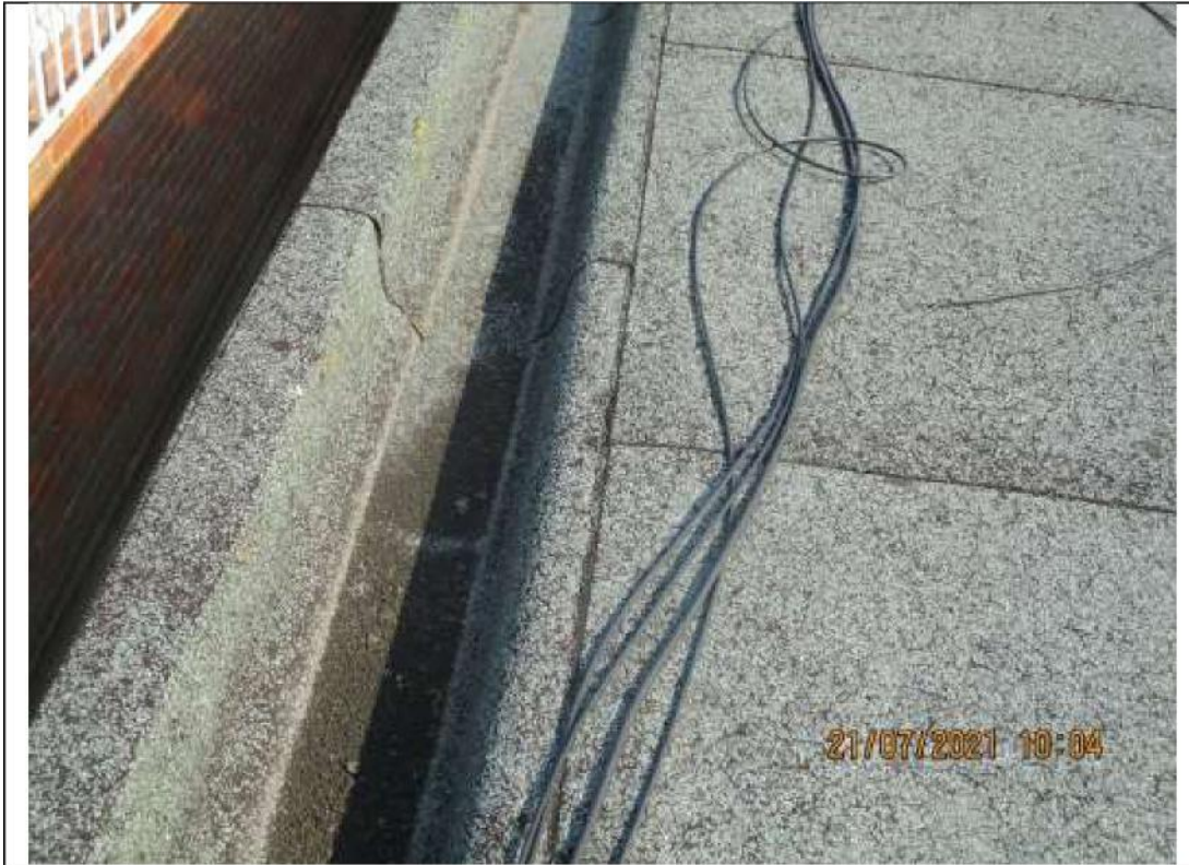
29) Link roof to gymnasium building.
