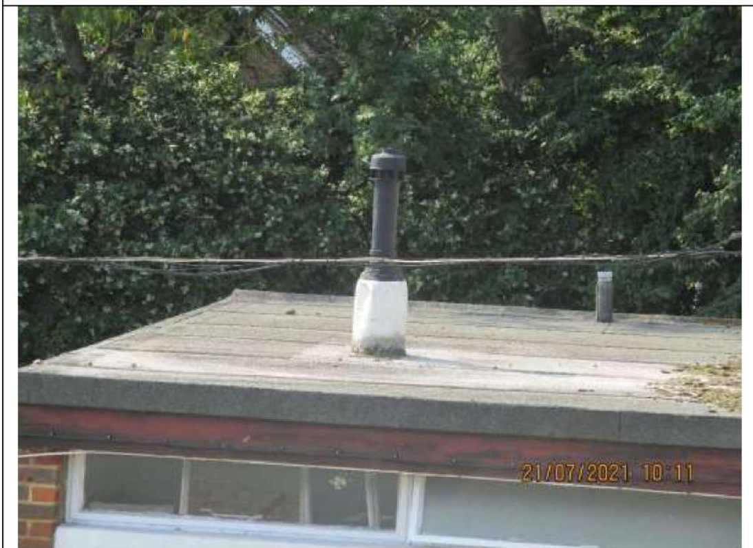
32) Flat roof above Year 5/6 block.
