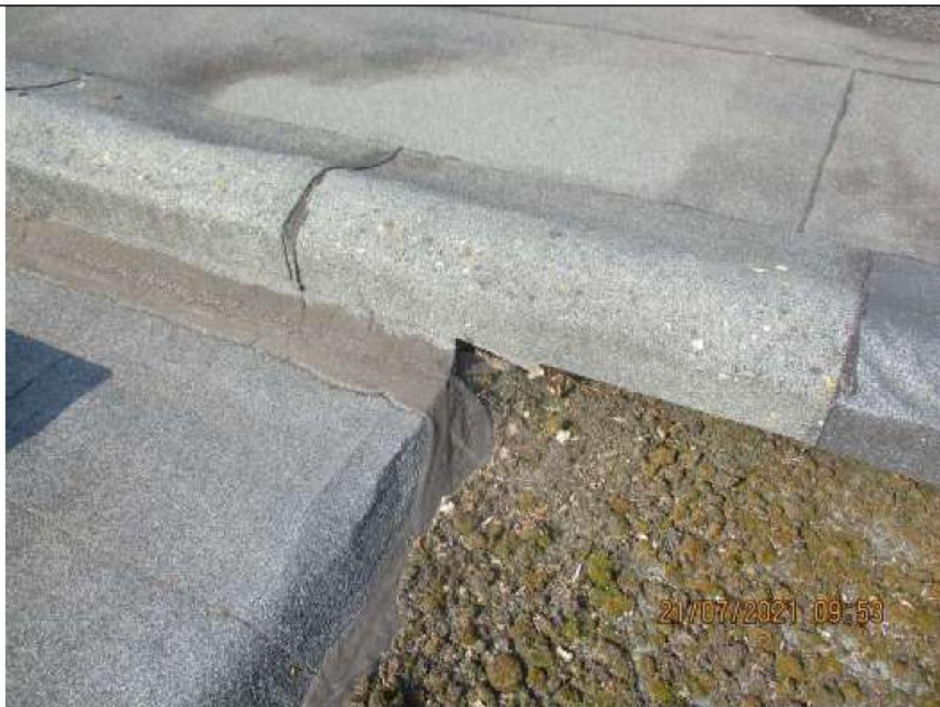
20) Patch repairs to roof above KS2 area.
