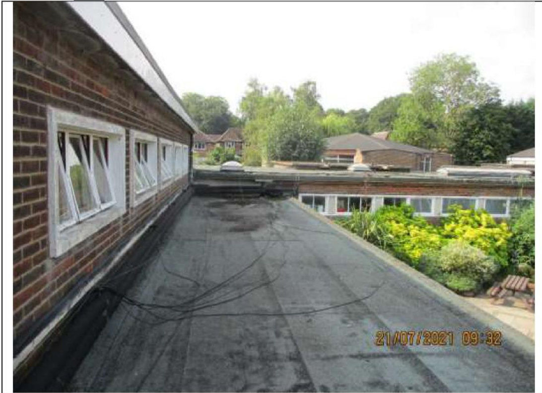
1) Lower level roof adjacent to the hall.
