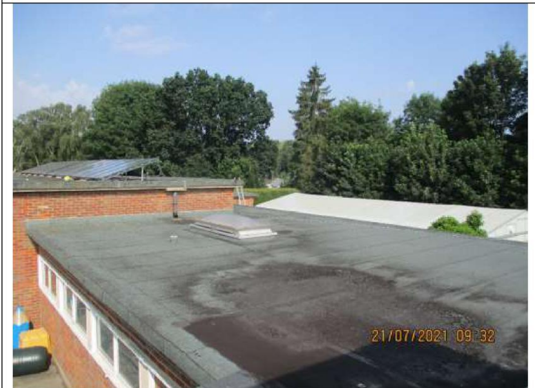
2) Flat roof above KS1 area.
