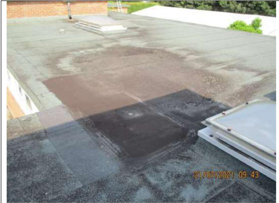
13) Patch repairs to flat roof area.
