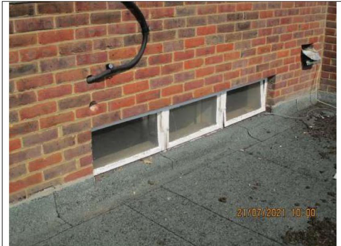
27) Low level windows to roof adjacent to the nursery.
