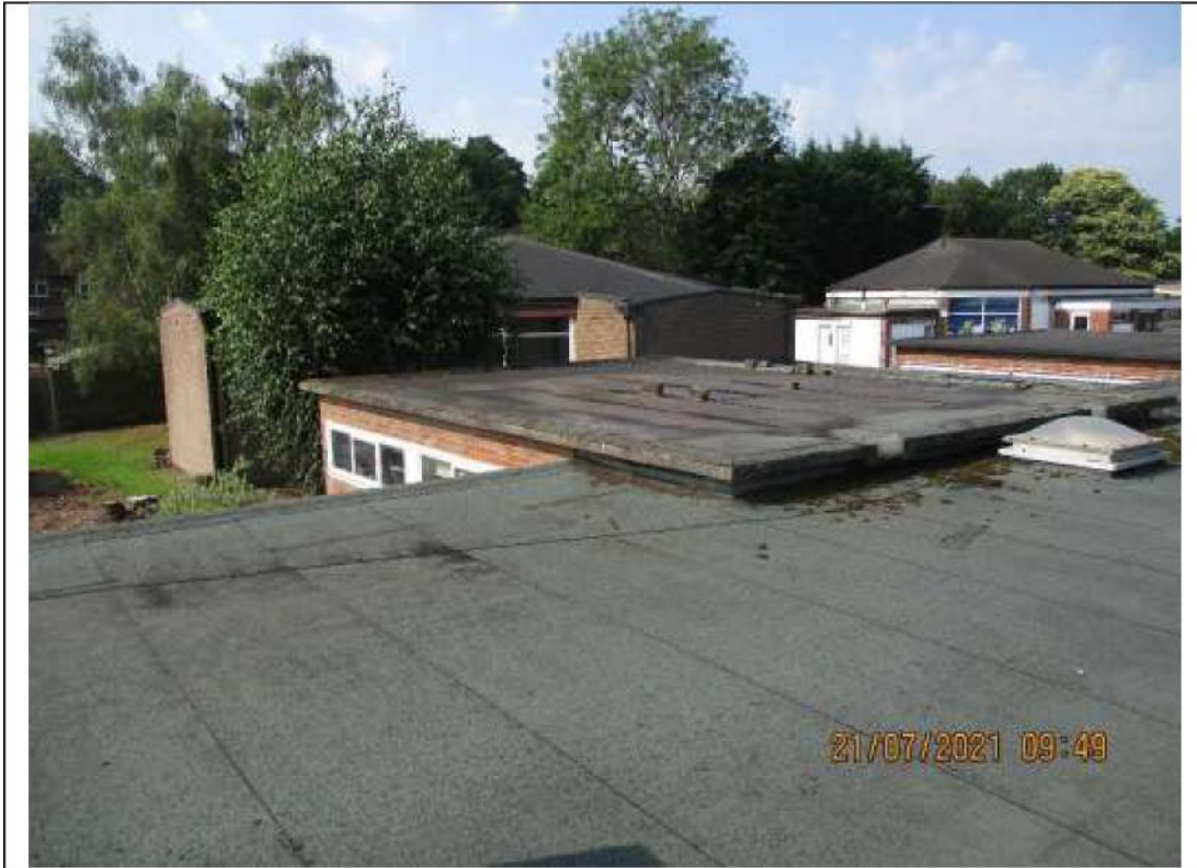
17) Roof above KS2 area.
