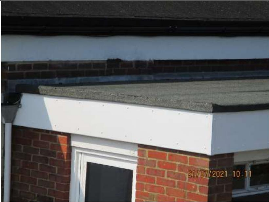
33) Flat roof above Year 5/6 block.
