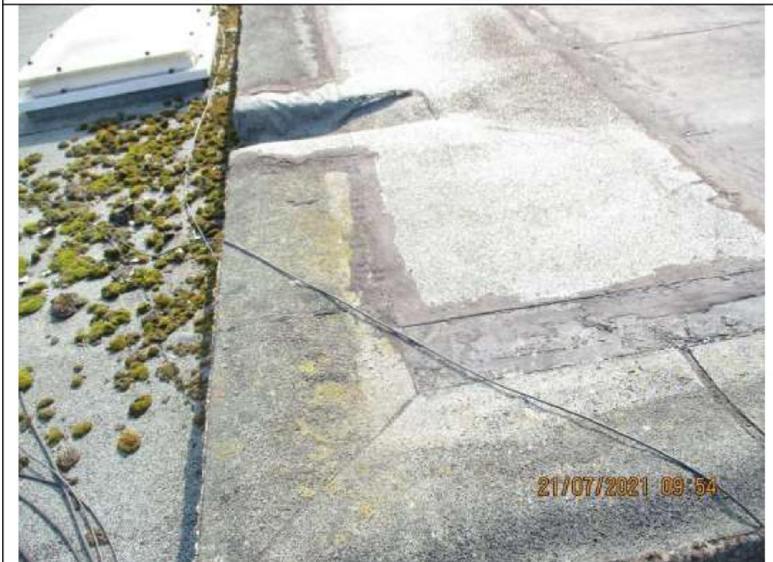
22) Patch repairs to roof above KS2 area.
