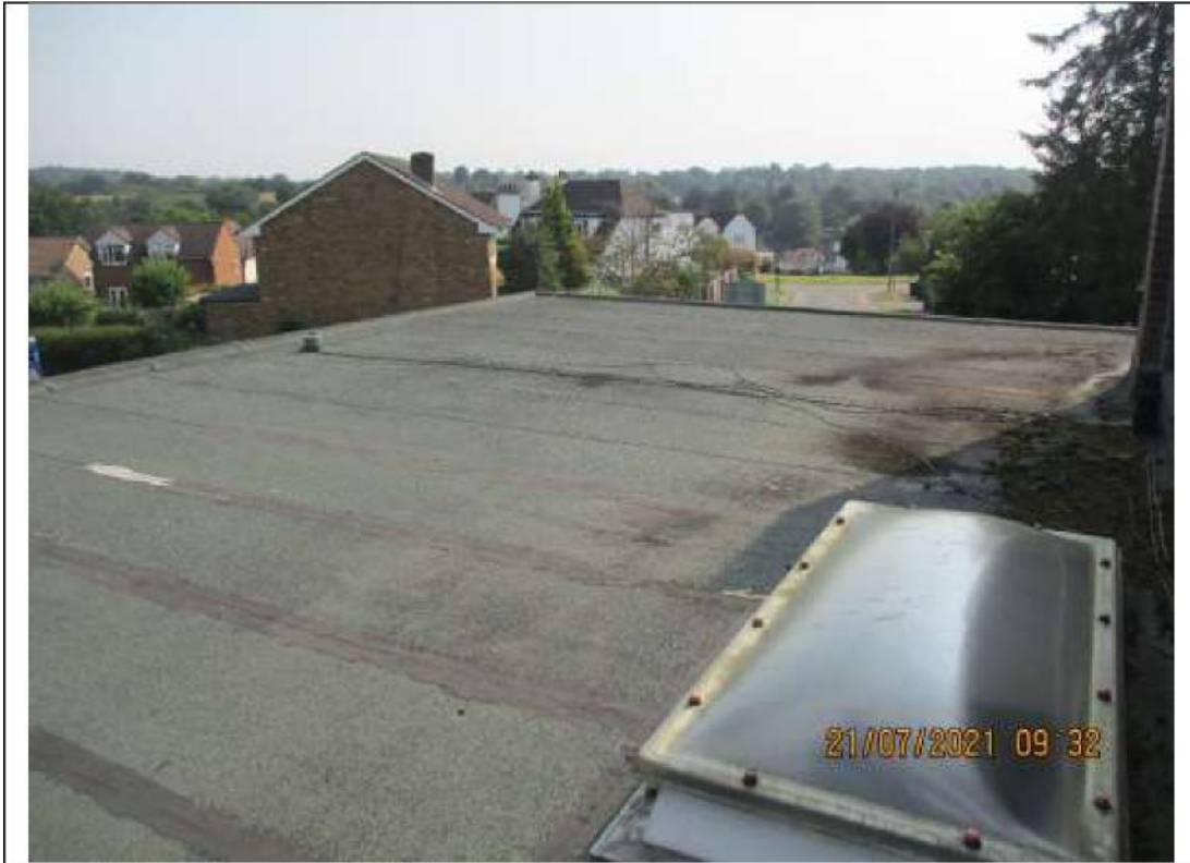
3) Flat roof above KS1 area.
