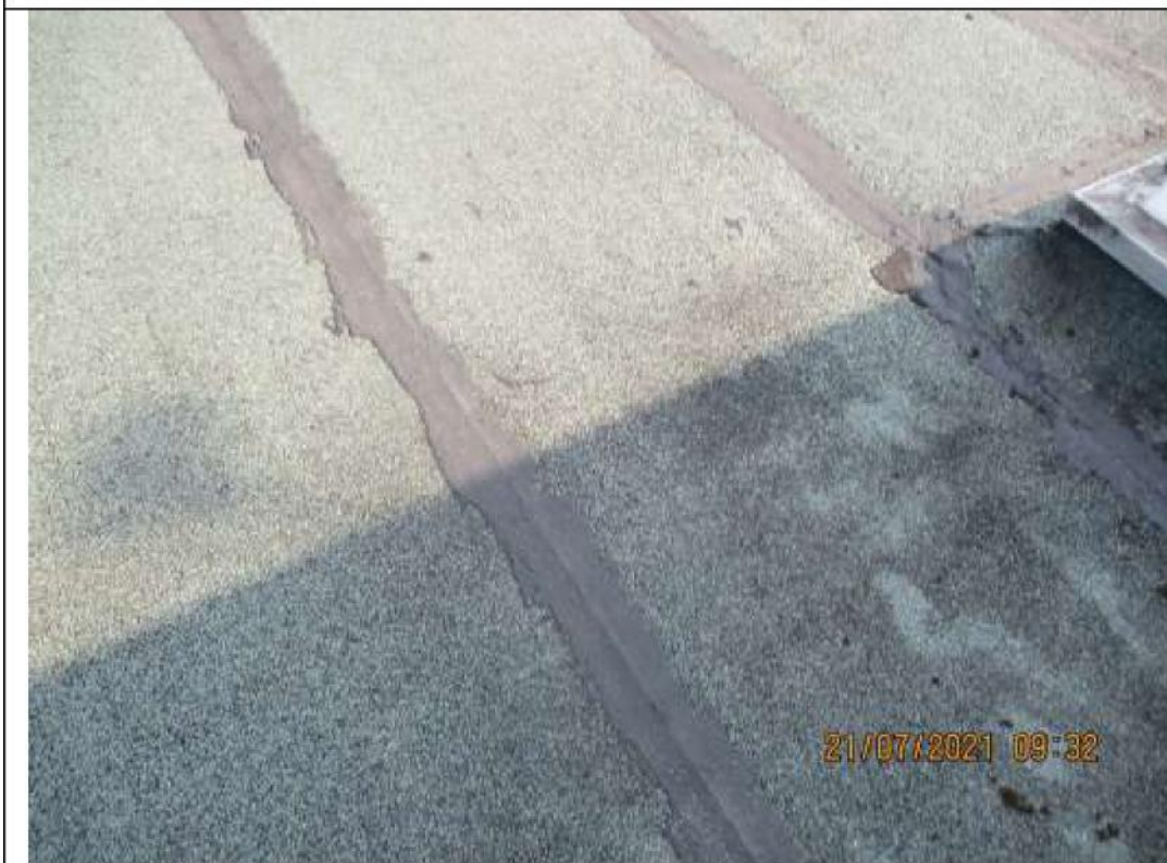
4) Temporary patch repairs to roof coverings.
