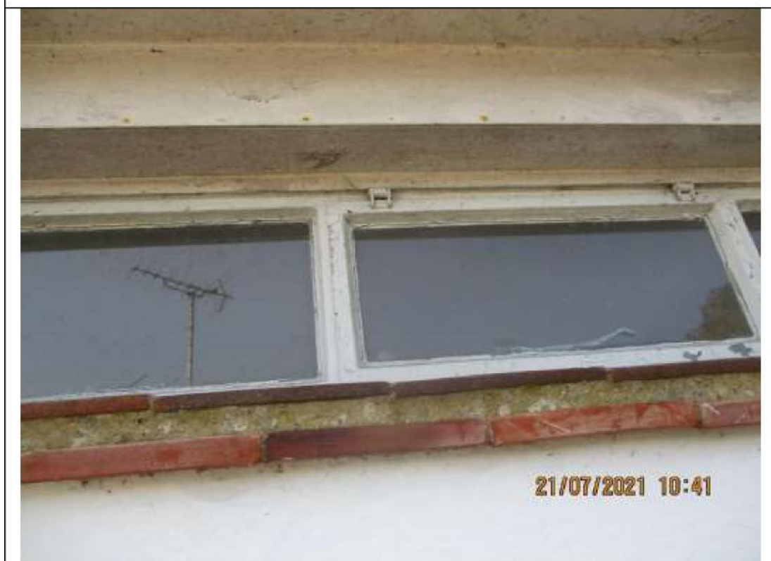
44) Single glazed windows to Year 5/6 block.
