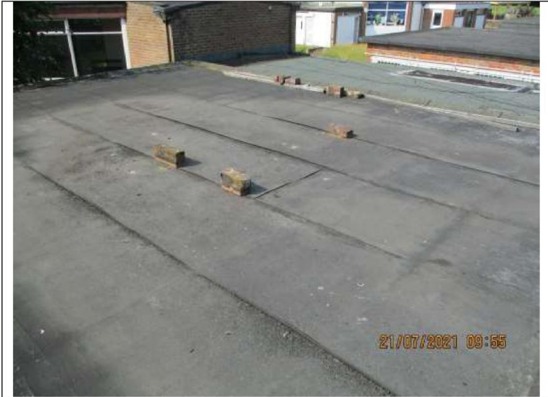
23) Patch repairs to roof above KS2 area.
